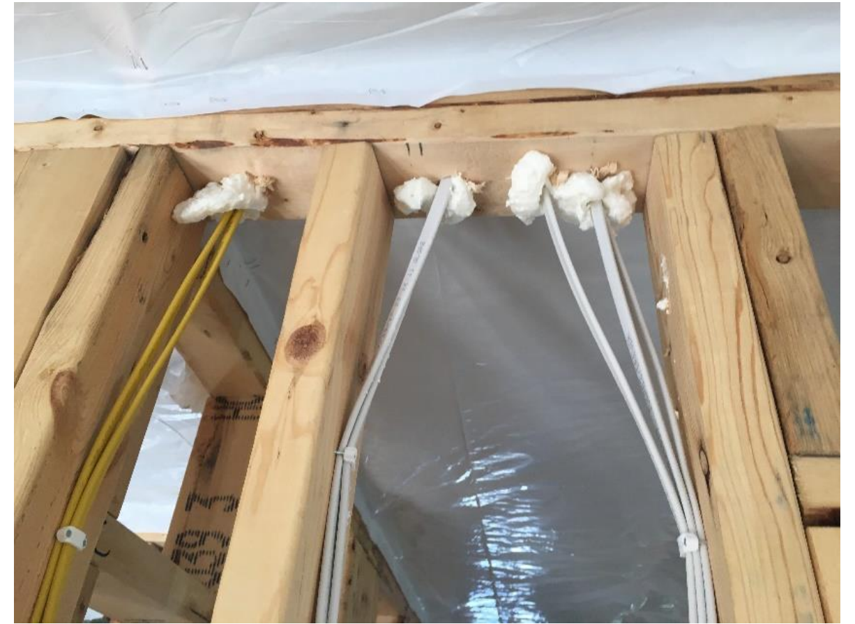
Can foam at wire penetrations
