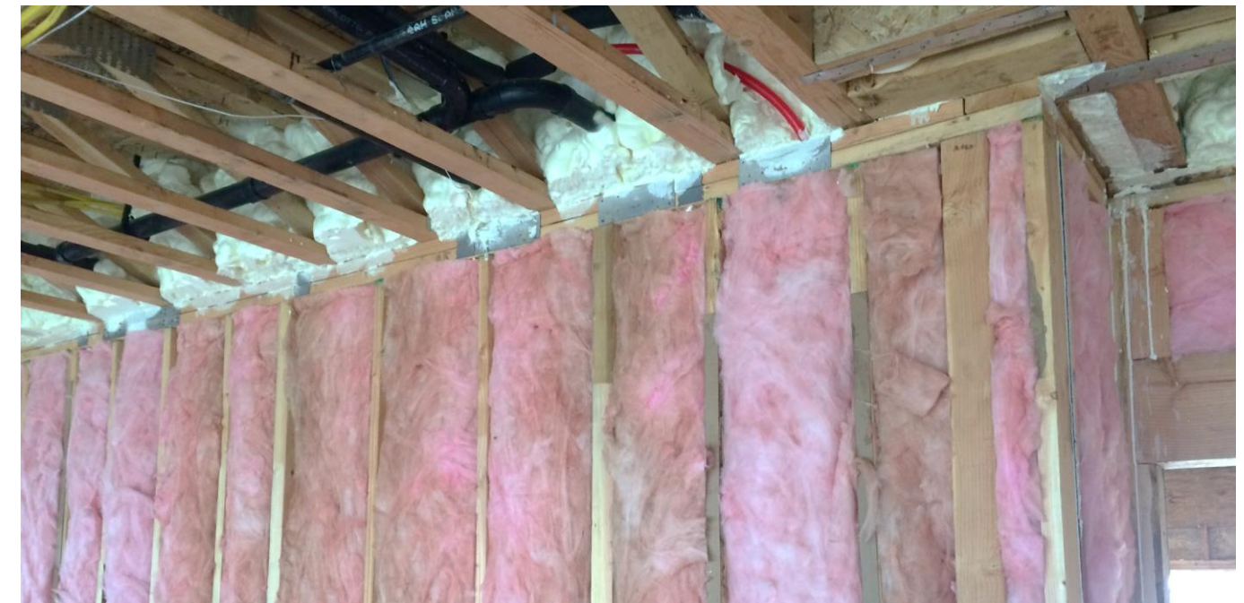
Foam at rim joist
