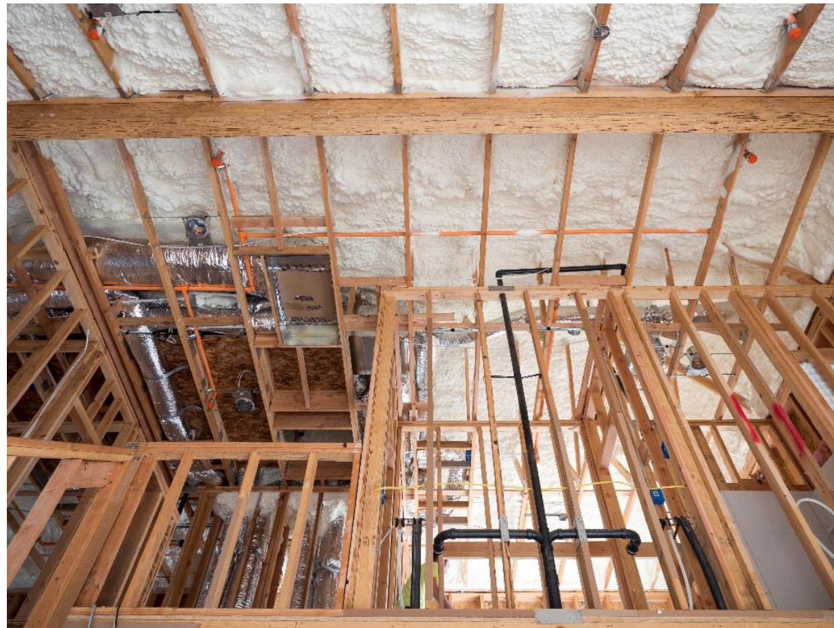
Foam at roof deck
