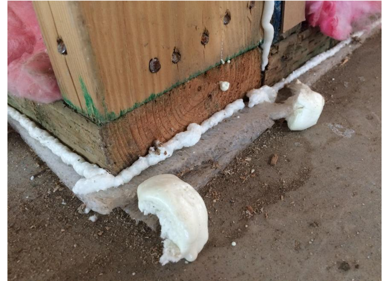
Can foam and gasket at sill plate
