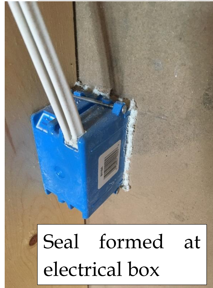
Seals formed at wire penetrations
