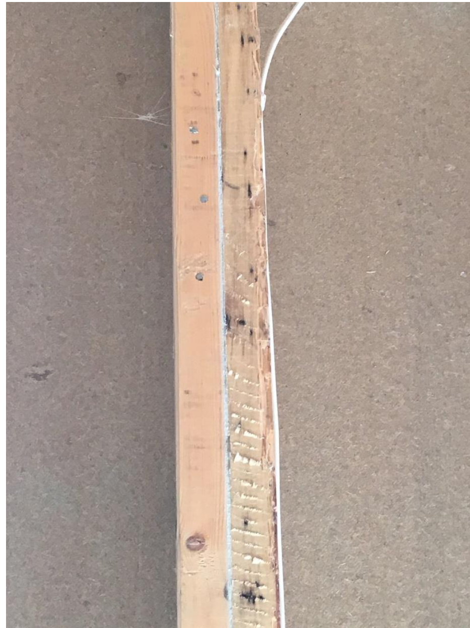
Seal formed between studs
