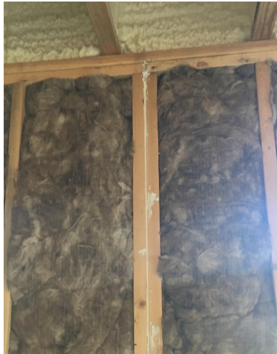
Caulk at seams where wood is joined
