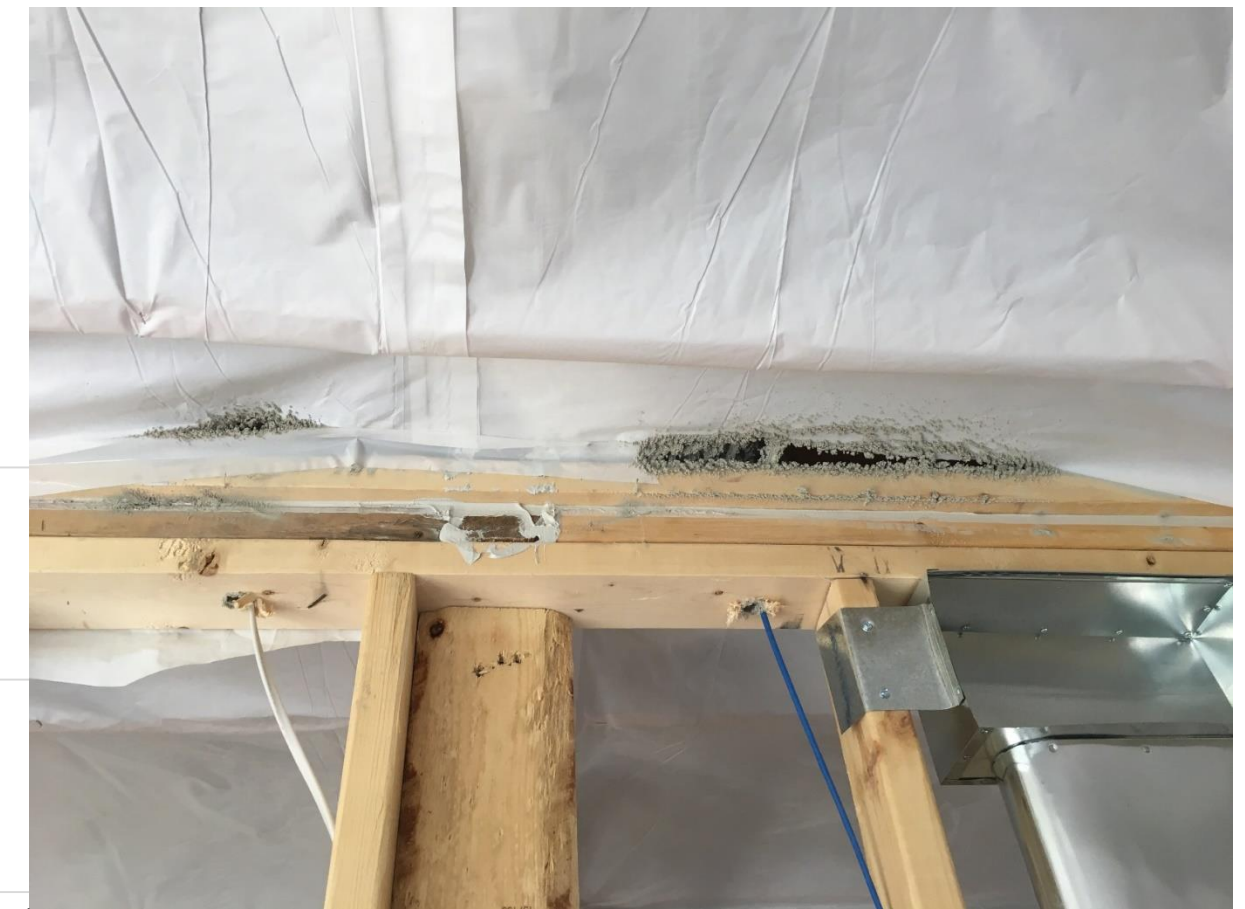
Reinforced poly failed
