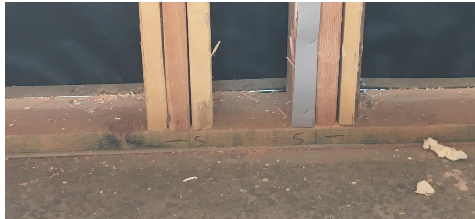
Foam gasket at sill plate
