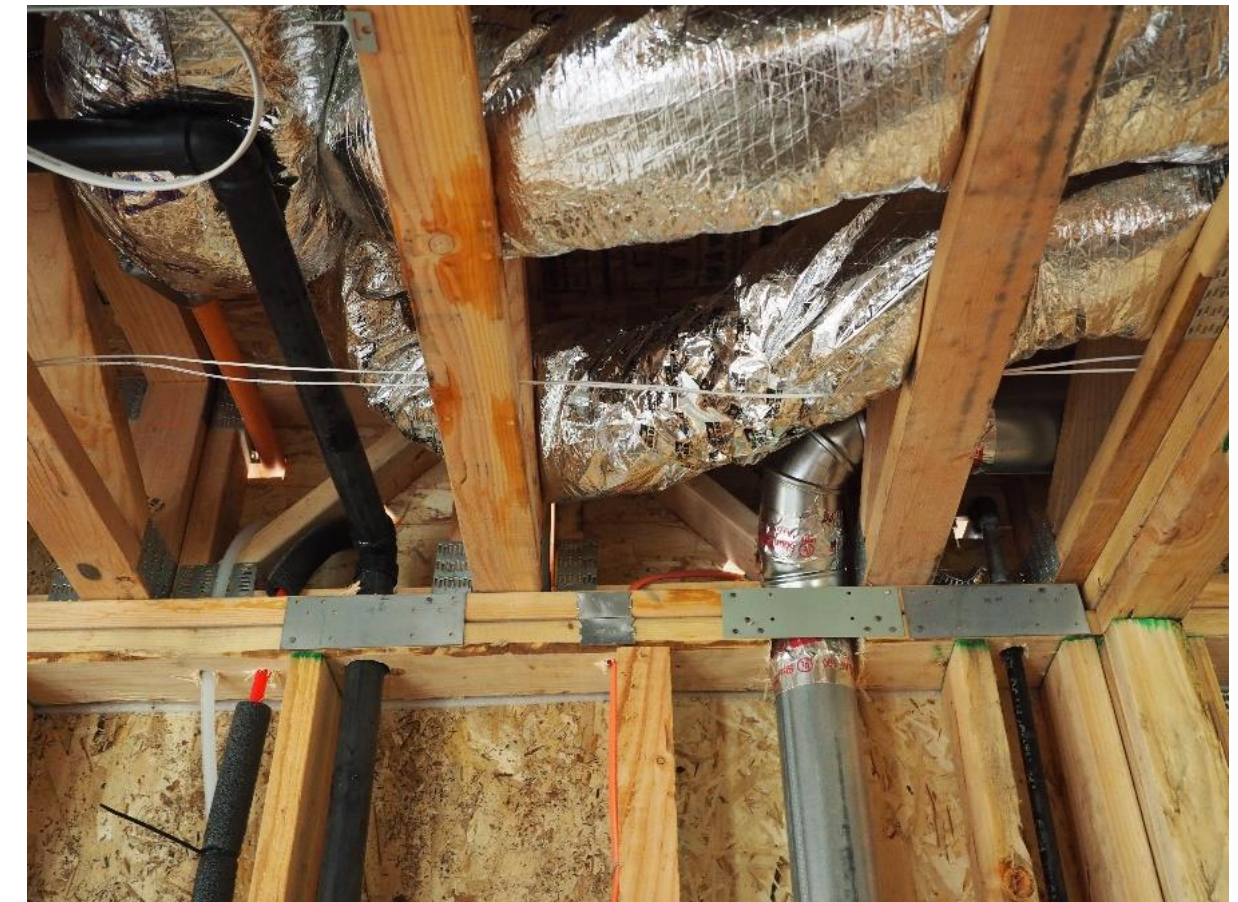
Rim joist penetrations
