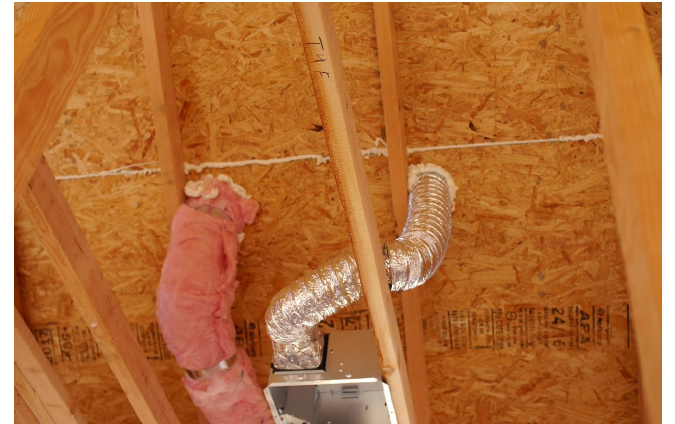
Can foam in expansion joint at roof deck and HVAC penetrations
