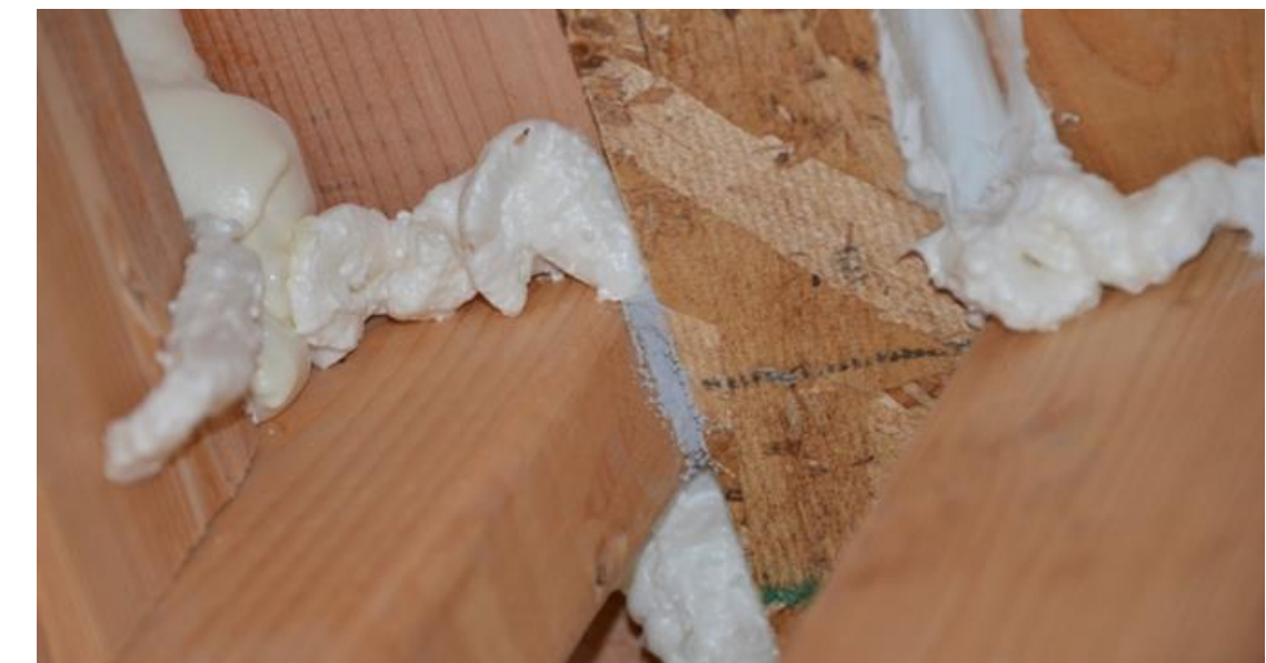
Seal formed between gap in foam
